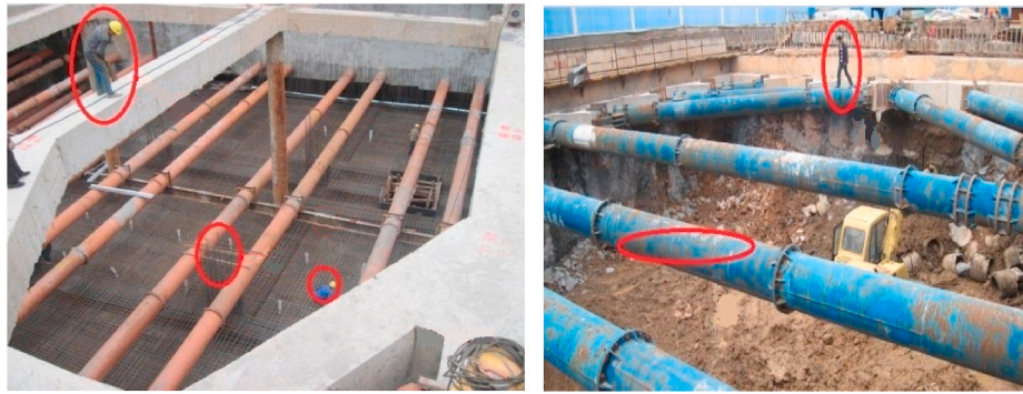
Fig. 8. Structural support for deep foundation pits.
